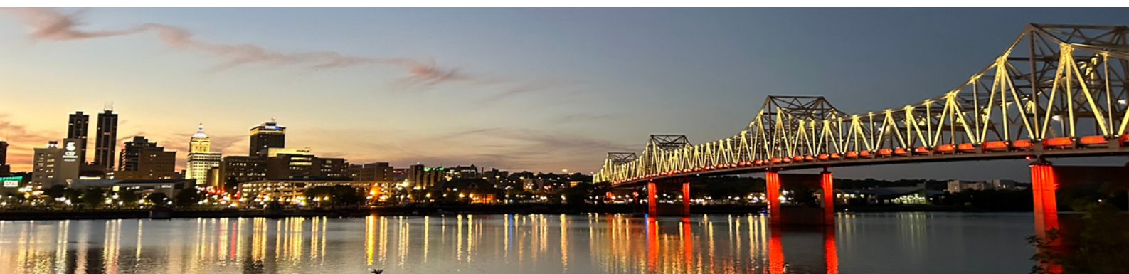
Bridge Illuminated Orange for Hunger on September 1st - Thanks to Peoria Area Food Bank & Midwest Food Bank
